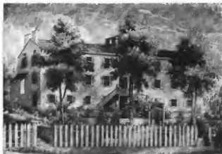
GROVE ACADEMY AND FORMER STEUBENVILLE HIGH SCHOOL
